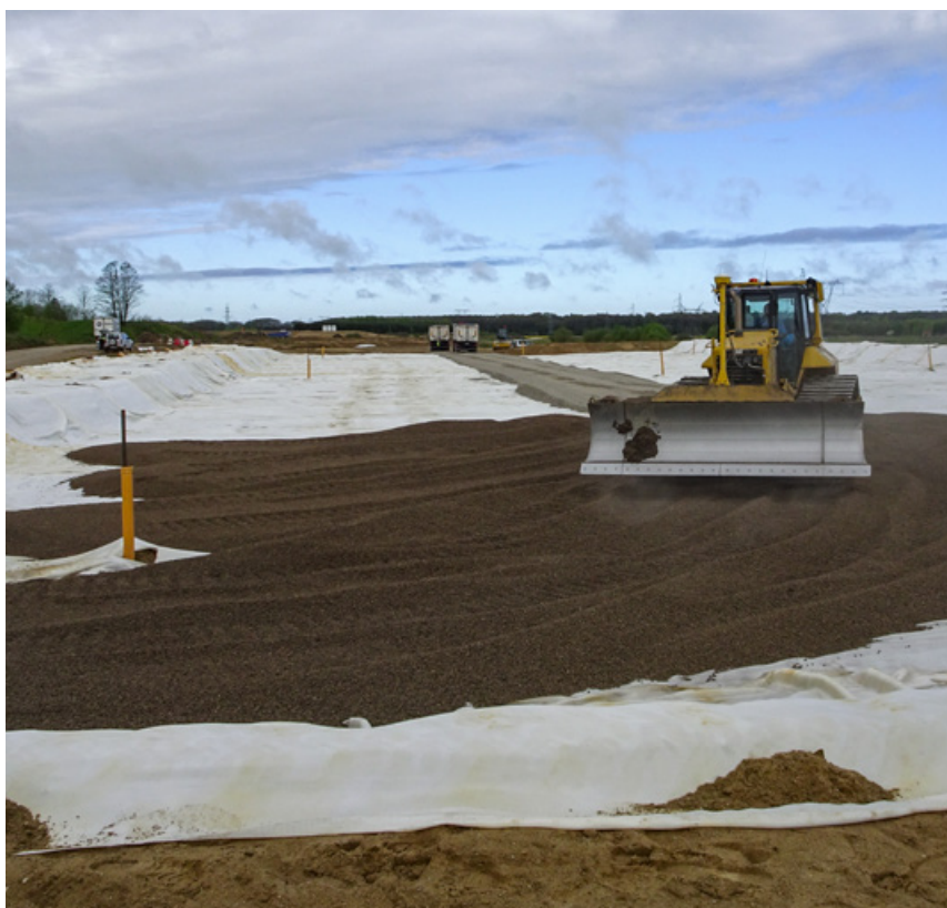
On three sections of the main route, mattress layers of Leca LWA (Leca® GEOTECHNICAL 8/10-20 RX) were designed and constructed
