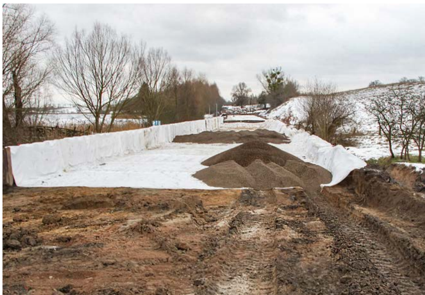
It was decided to use a geomattress made of Leca® GEOTECHNICAL EXPANDED CLAY 8/10-20RX.”
