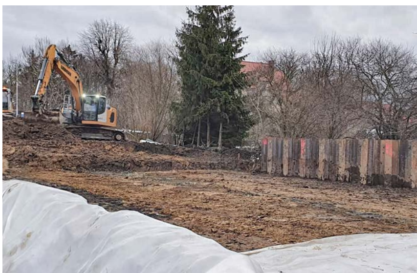
A protection of the track bed crown was constructed in the form of a retaining structure made of a sectionally anchored steel sheet pile wall.
