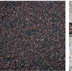
**The gaps** between the paving stone were filled with crushed Leca LWA to ensure unobstructed water flow.
