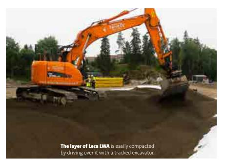
"The project uses almost 8000m3 of Leca Lightweight Aggregate (LWA) as a lightweight filling for improving the Klaukkalantie road, as well as the construction site of a new travel centre." says Site Manager Mikko Parkkinen, the project's main contractor for Graniittirakennus Kallio Ltd.
