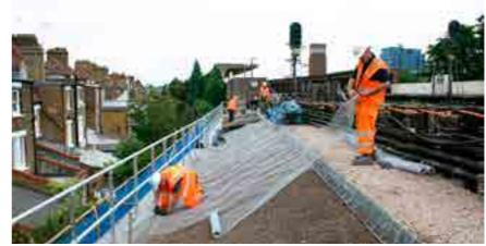
Deterioration of the embankment was compromising the stability of the wall alongside a busy station.
