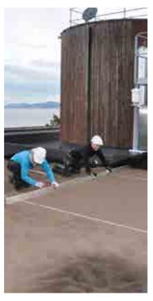
The fine Leca water detention material was levelled by plank and was not mechanically compacted.
