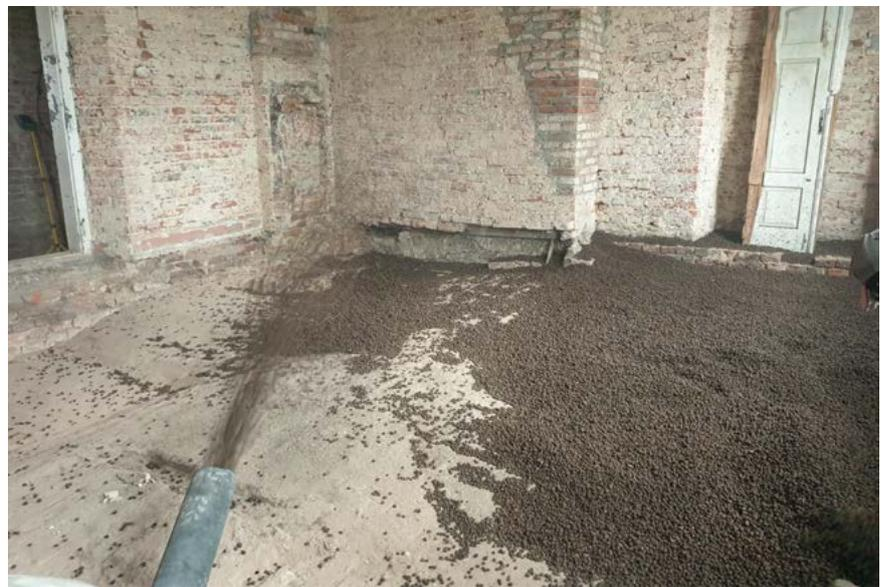
**Aggregate laying with** the use of a pump.
