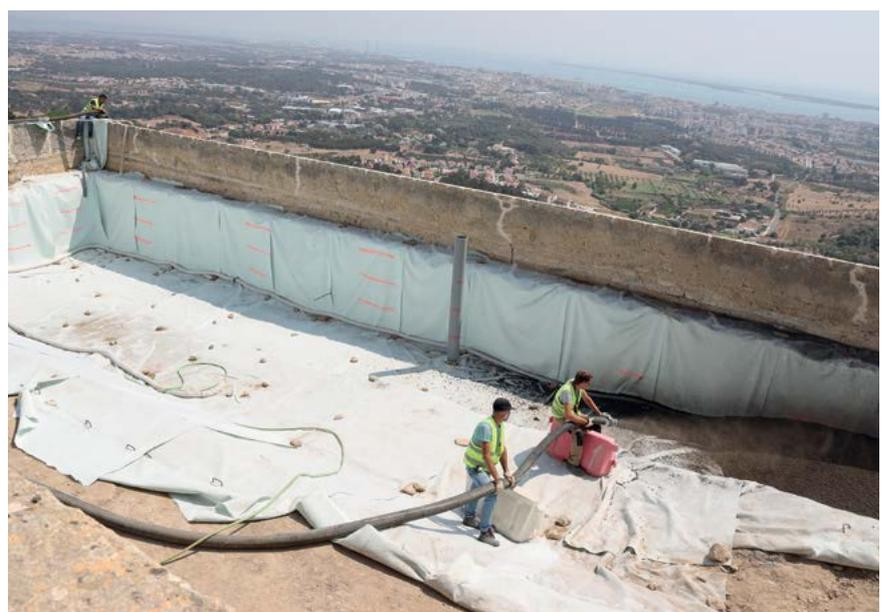
Leca LWA was pumped directly through pneumatic delivery.
