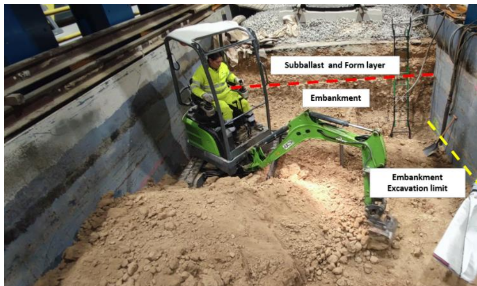
Figure 22.- Excavation of the embankment using machinery
