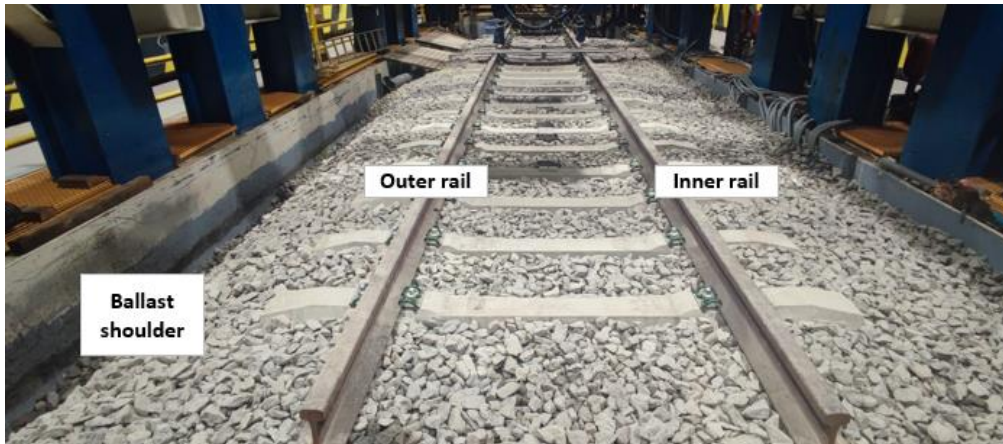
Figure 15.-Ballast layer used in the railway track section
