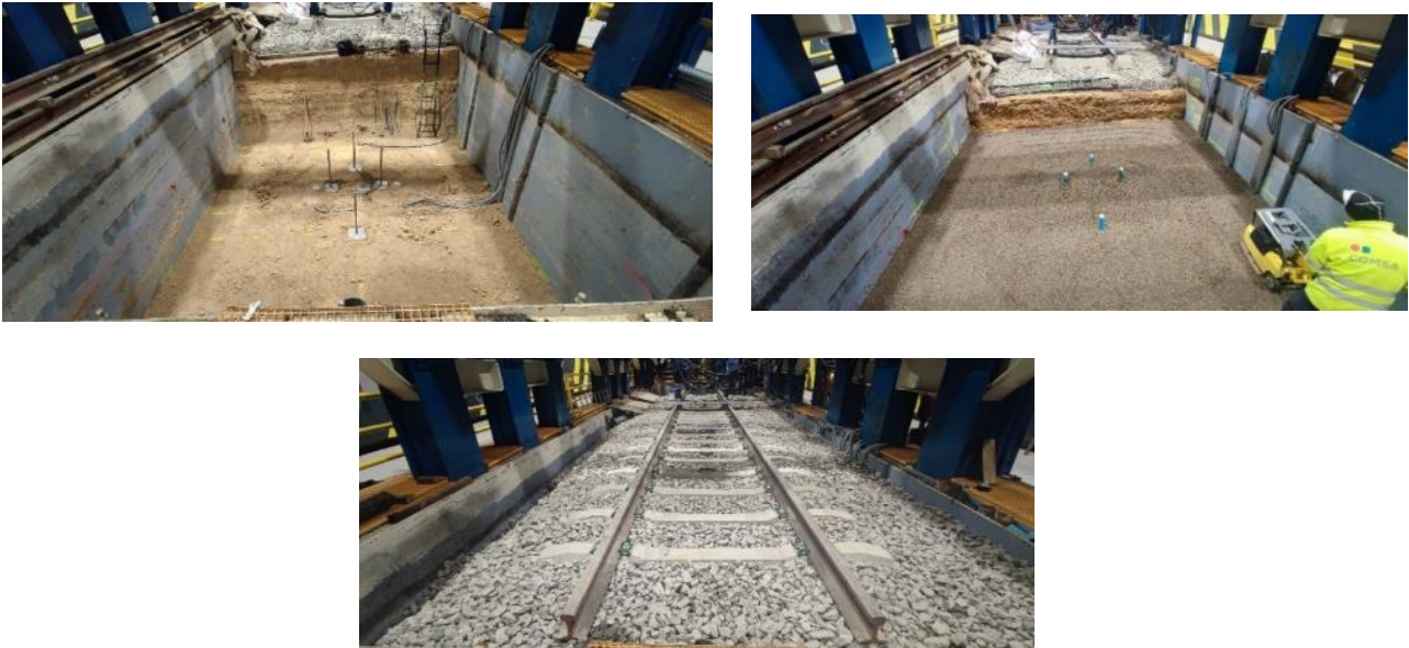
Figure 3. Different stages of model construction. Top left: embankment excavation completed. Top right: LECA embankment during compaction. Bottom: PEDLER railway track test section finished.
