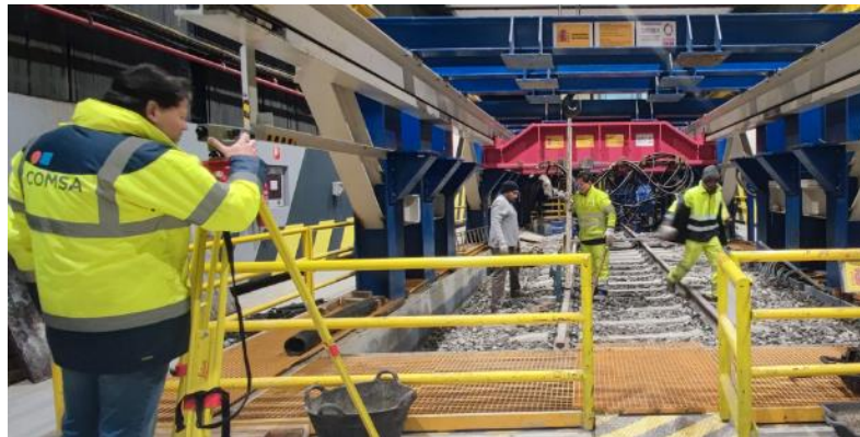
Figure 44.- Levelling of railway track sections.
