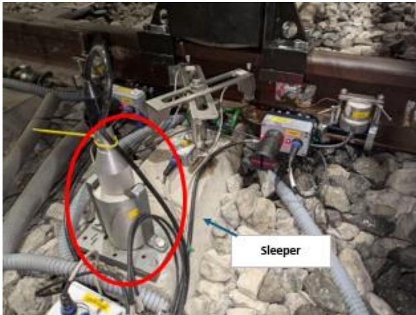
Figure 55.- Geophone located at sleeper
