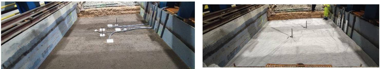
Figure 33.- Left: LECA embankment top with instrumentation. Right: Geotextile over LECA embankment
