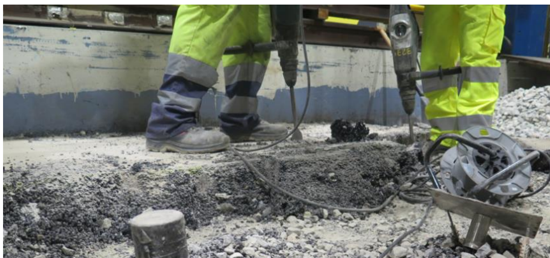
Figure 20.- Dismantling the foundation layer of the previous test
