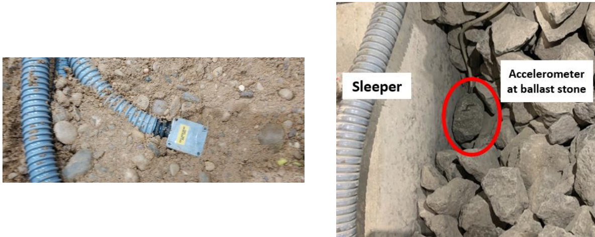
Figure 49.- Example of an accelerometer installed inside the railway track section (left) and instrumented ballast particle (right)
